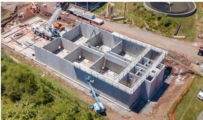
Erection of precast sections of the rectangular activated sludge basin at Upper Montgomery Joint Authority WWTP in Pennsburg, PA (Photo courtesy Dutchland, LLC)
