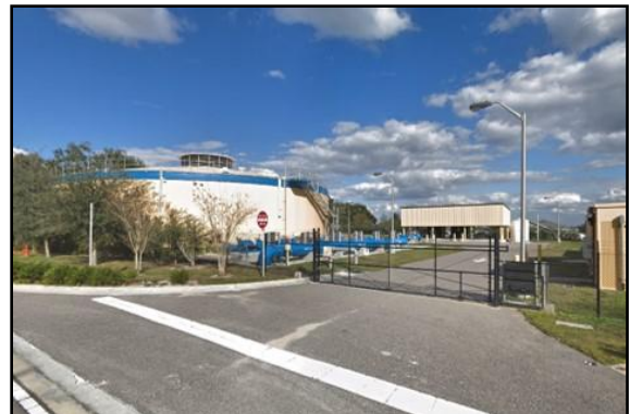
Pollard Road Water Treatment Facility
