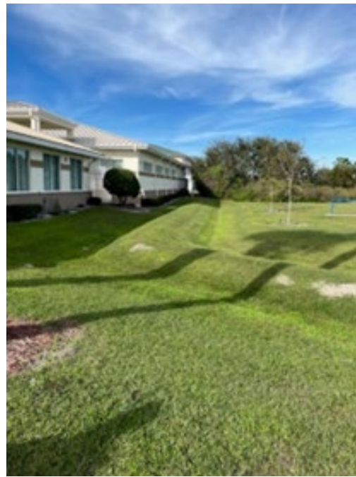
Figure 26: Site Drainage Swales
