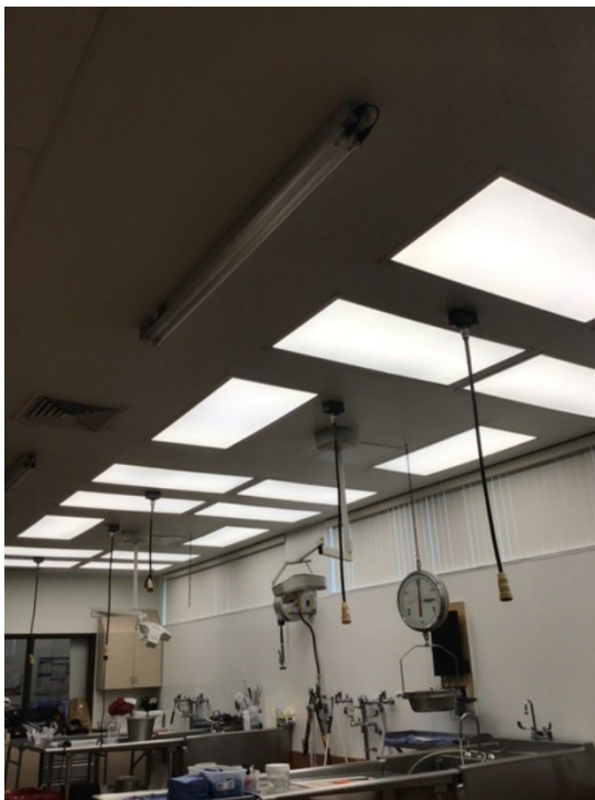
Figure 33: Autopsy Lab Lighting and Power Drops
