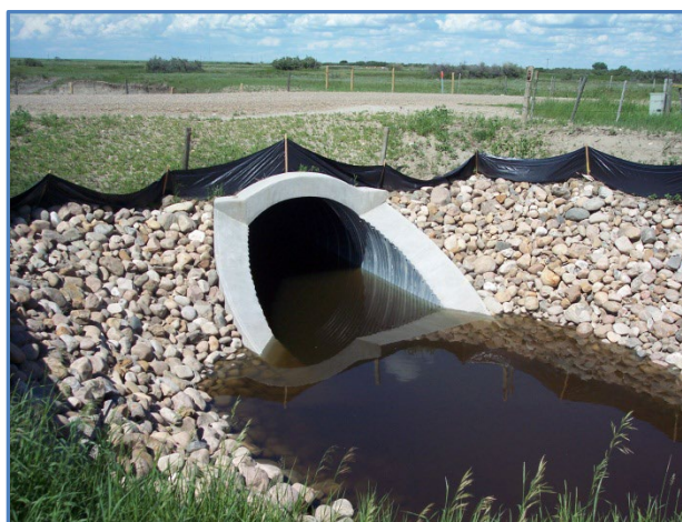
Figure VII.9: Culvert modifications
