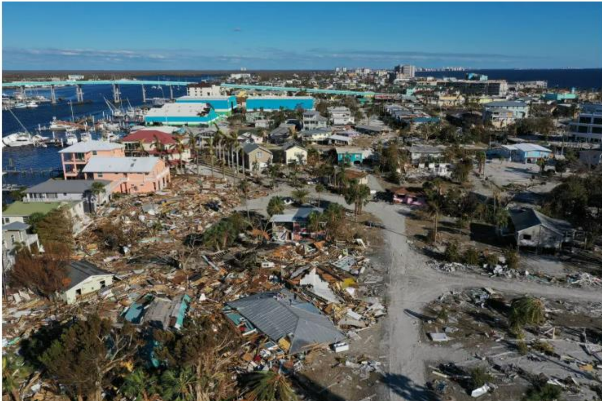
FORT MYERS BEACH, FLORIDA – OCTOBER 02: In this aerial view, destruction left in the wake of Hurricane Ian is shown on October 02, 2022 in Fort Myers Beach, Florida. Fort Myers Beach sustained severe damage by the Category 4 hurricane which caused extensive damage to the southwest portion of Florida. (Photo by Win McNamee/Getty Images)
