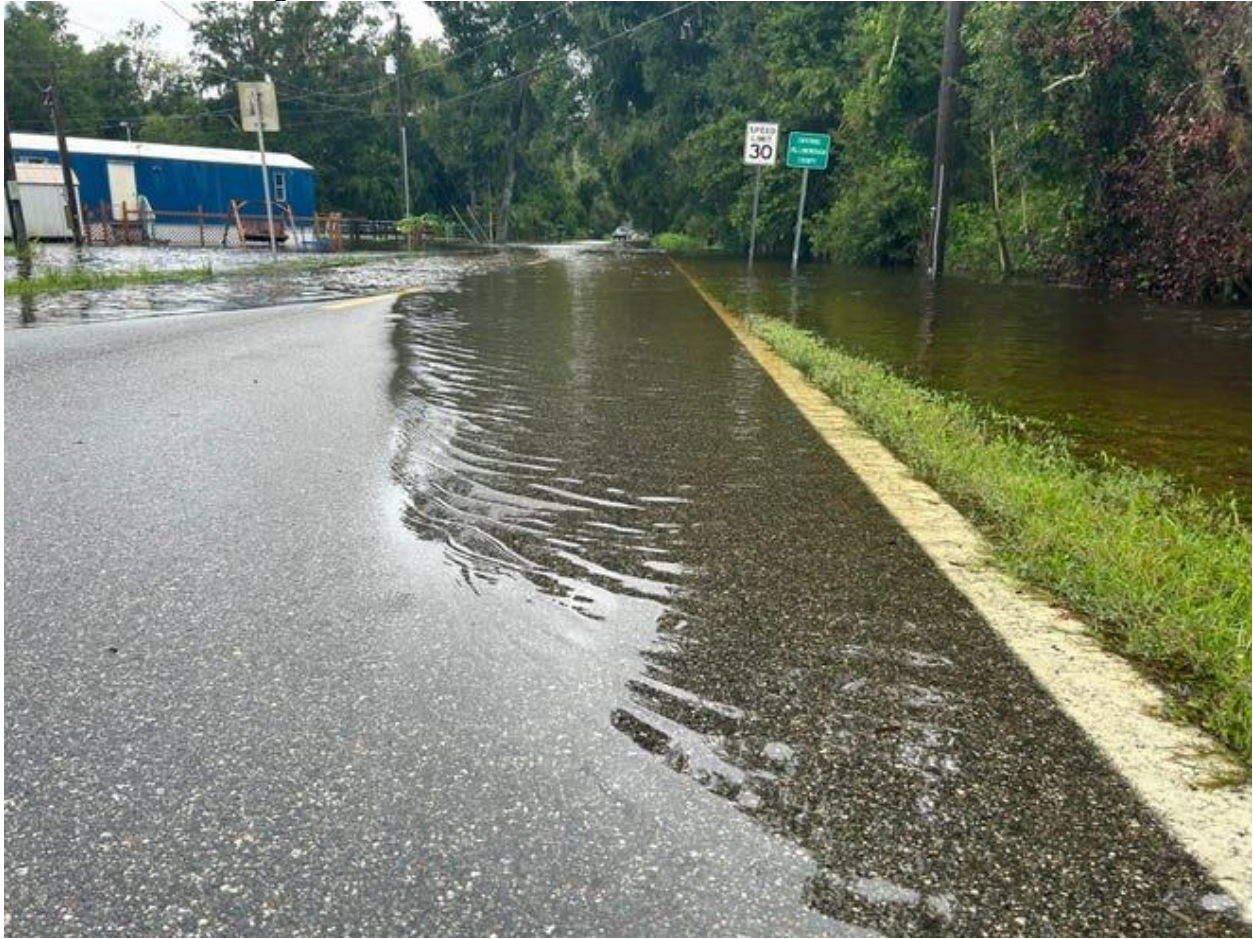
Flooding along Deeson Road in Kathleen due to Hurricane Debby Andy Kuppers
