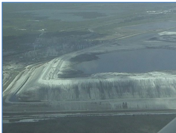
Figure V.38: View of a phosphogypsum stack. Source: www.fluoridealert.org
