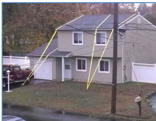
Figure VII.10: Tie-downs for windproofing
