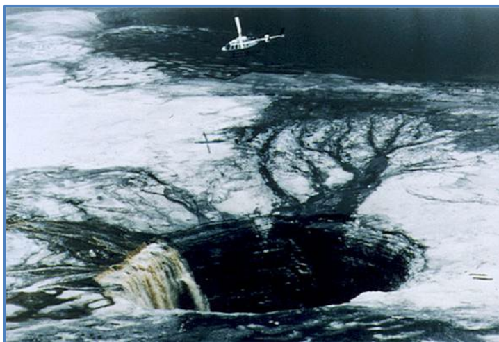
Figure V.39: Sinkhole in Center of IMC-Agrico Waste Stack Near Mulberry, June 1994 Source: www.fluoridealert.org (AP Photo)
