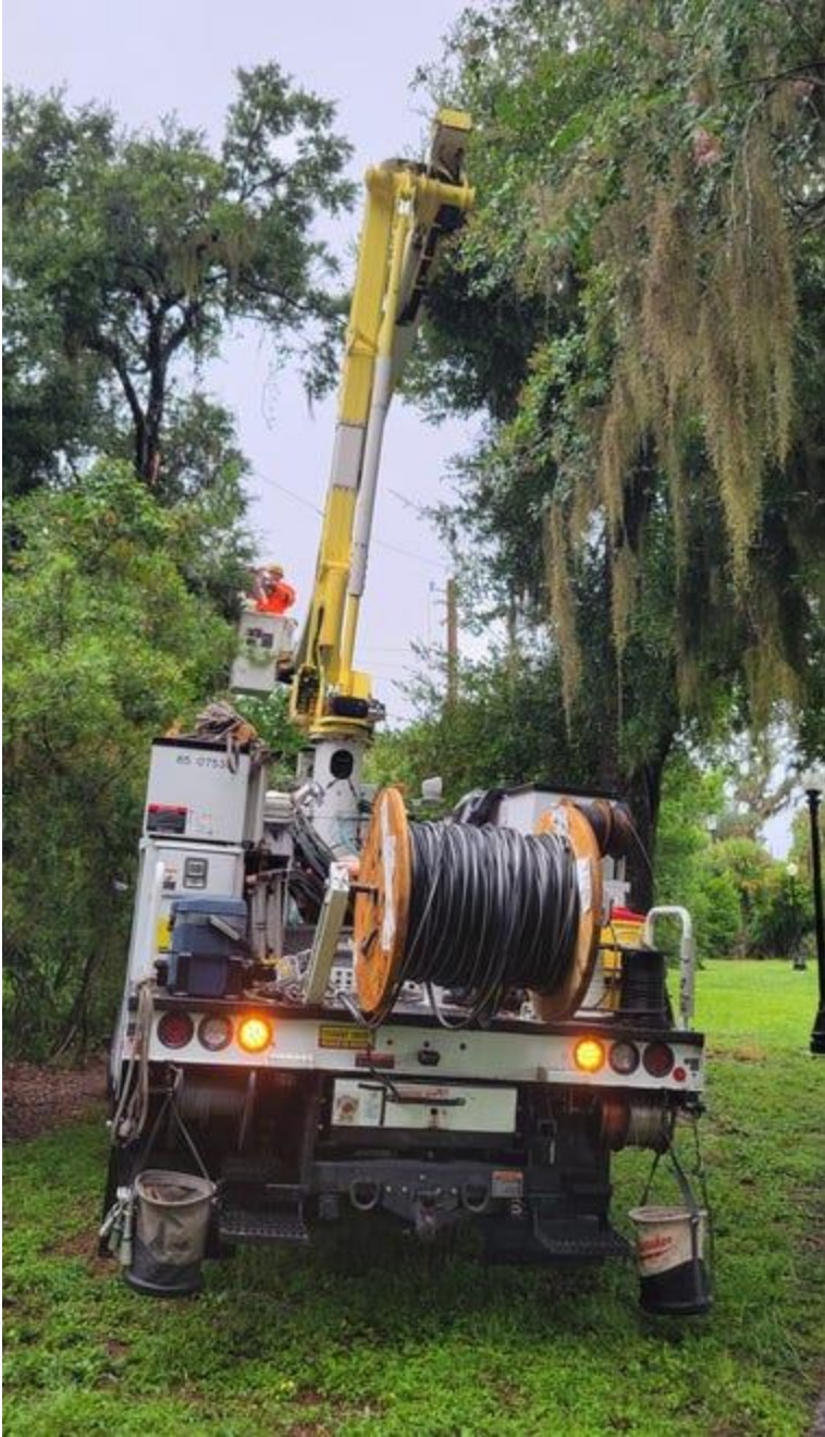
Electric crews restoring power in Polk County due to Hurricane Debby.
