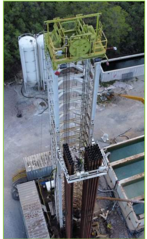
LFA deep-well drilling rig
