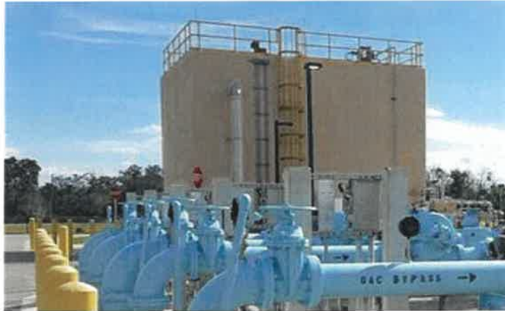
Photo 2. The ozone contact and destruct chamber
