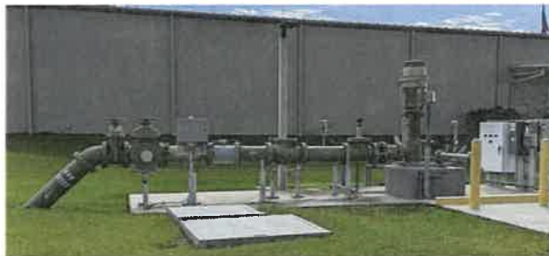
Photo 1. One of three Central WTF On-site Wells.
