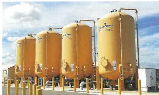
Photo 3. Central WTF Adsorber GAC Adsorption Vessels
