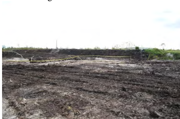
Pile G facing Southwest
