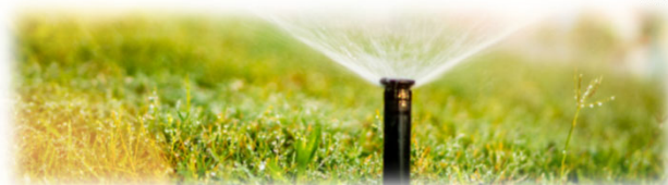
a minimum of 6-inch pop-up for sprays and 4-inch pop-up for rotors for St. Augustine, Zoysia and Bahia grasses.
