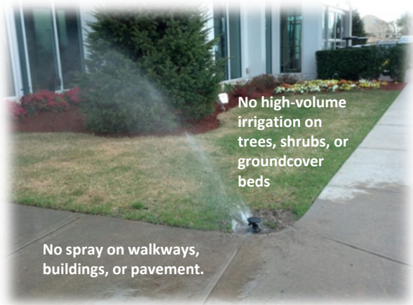
a minimum of a 4-inch pop-up for sprays and rotors for Centipede, Bermuda and Seashore Paspalum grasses
