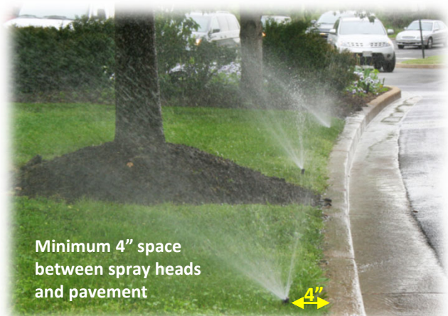
a minimum of 6-inch pop-up for sprays and 4-inch pop-up for rotors for St. Augustine, Zoysia and Bahia grasses.
