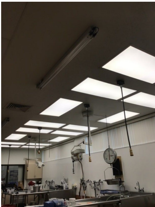
Figure 33: Autopsy Lab Lighting and Power Drops
