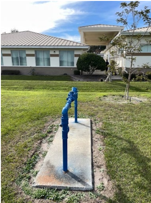
Figure 25: Water Service/Backflow Preventer
