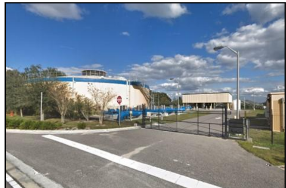
Pollard Road Water Treatment Facility
